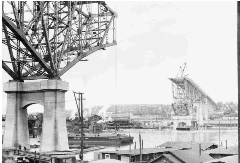
Figure 7: Floating Homes on Lake Union, 1931
