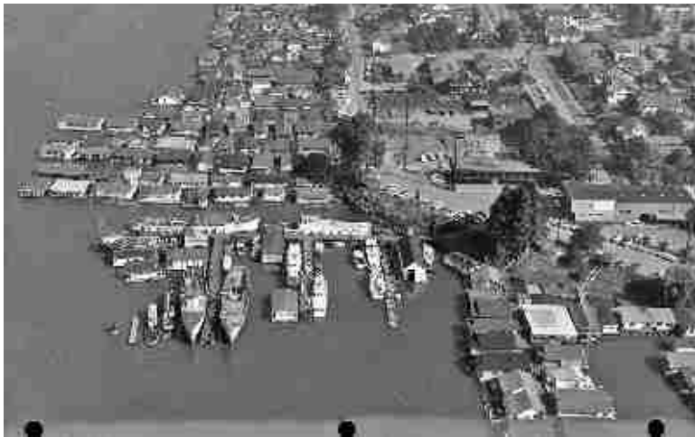
Figure 6: Floating homes on Lake Union, 1962.
